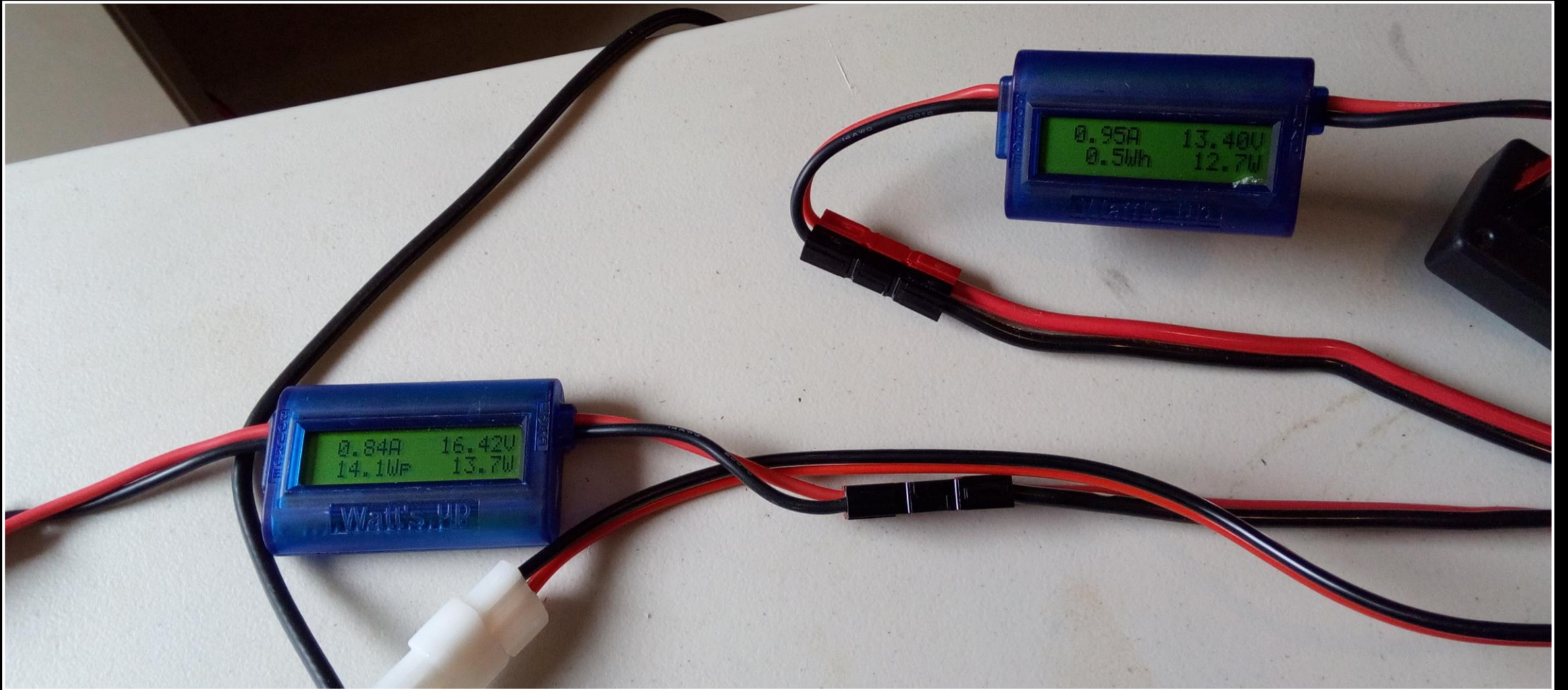
CLOUDY SKY WITH 120 WATT SOLAR AND GENASUN GV-10 MPPT CHARGE CONTROLLER, PANEL INPUT IS LEFT WATTS UP METER
