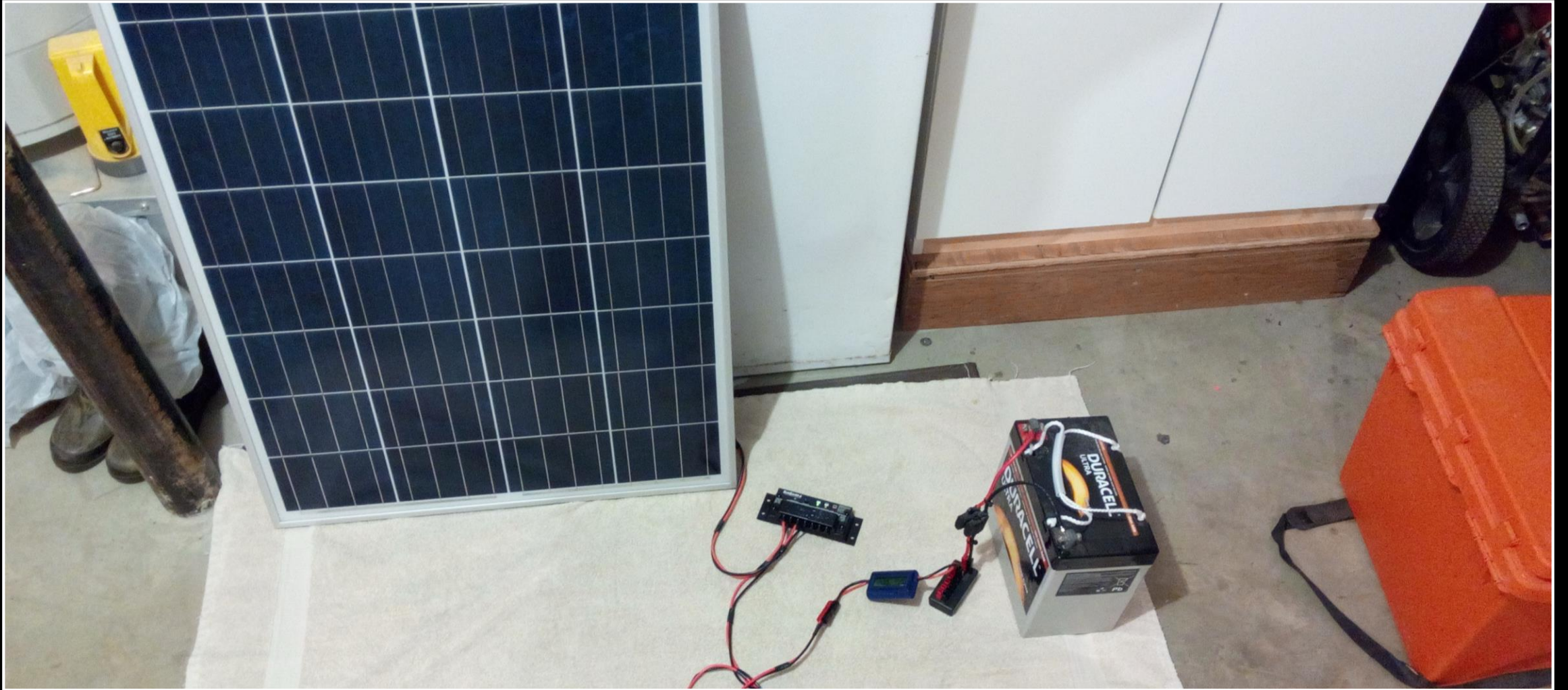
SYSTEM #2 IS A RENOGY 100 WATT SOLAR PANEL AND MORNINGSTAR SUNSAVER 6 CHARGE CONTROLLER WITH DISTRIBUTION BLOCK AND METER
